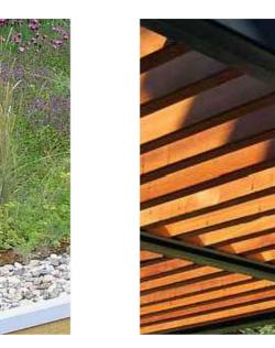
**07** - vertical timber slat canopy set into dark grey metal frame to match glazing system
