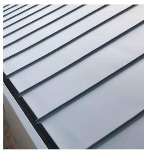
**05** - Zinc (or equiv) standing seam roof cladding with integral concealed gutter in Dark Grey
