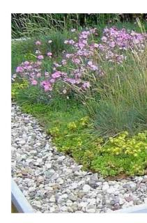
**06** - Sedum roof with gravel perimeter drainage and internal drainage
