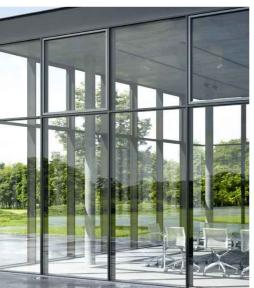
**03** - Schueco FWS50 Aluminium glazing facade system or eqiv. in dark grey with solar control double or triple glazing. Frame system target u-value of 0.9W/m<sup>2</sup>K or better
